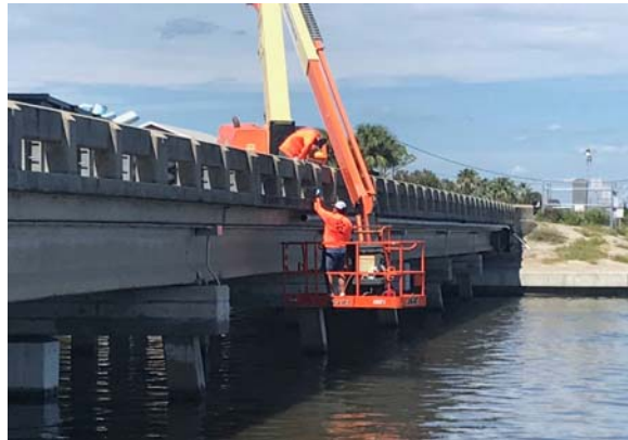
Pipe Removal From Bridge 3
